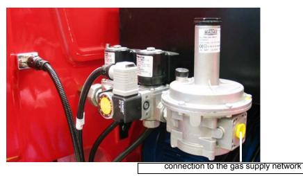
Once the gas train in installed, execute the electrical connections for all its items (gas valves group, pressure switch).
