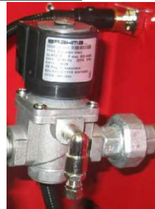
connection from the pilot gas train to the gas valves group of the main train
